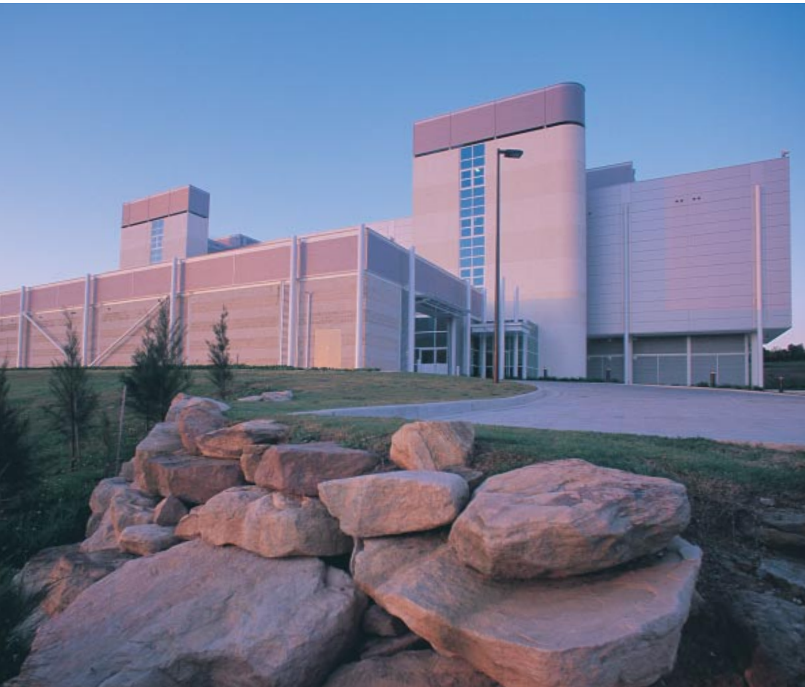
Client: Cathay Pacific. Architect: Woods Bagot. Structural Engineer: Connell Wagner. Panel Manufacturer: HH Robertson. Product: Formawall® Skin: COLORBOND® Metallic steel. Completed: 1996.
